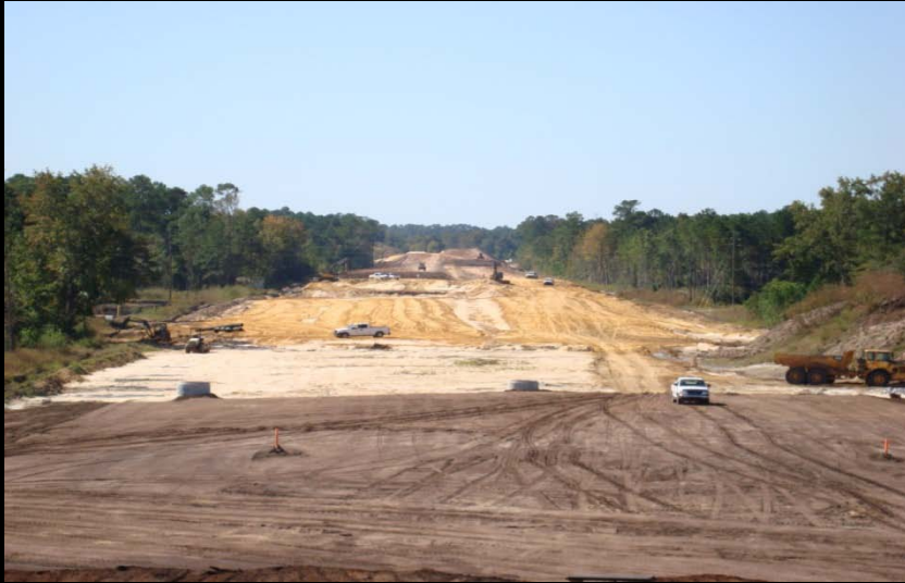
Early Clearing and Grubbing- Spring 2011
