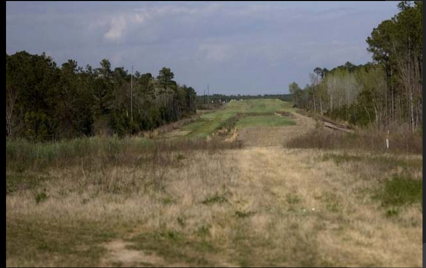
Early Clearing and Grubbing- Spring 2013
